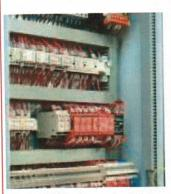
The logic blocks control the right working of the two safety channels, preventing unforeseen machine re-starts, or after power cut.
